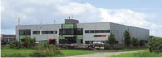
The new workshop that has cost NOK 70 million.
